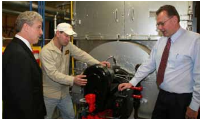
Ray Macco, Local 94 School Delegate with Jory Grief, and Custodian Engineer Bill Cunningham inspecting a boiler
