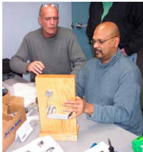
Students John McDermott and Jainarine Loutan install the cylinder and lock
