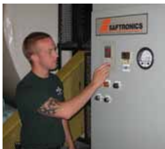
Jason Bowers adjusting a supply fan VFD
