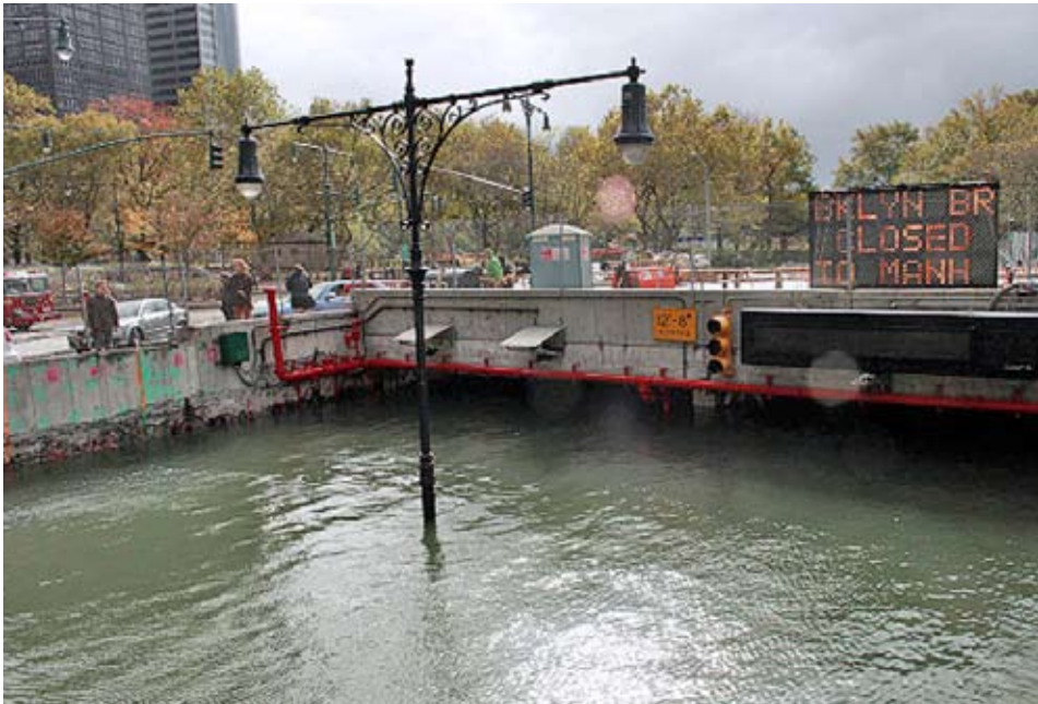
The Brooklyn Battery Tunnel was flooded with about 12 feet of water after a tidal surge caused by Sandy, Oct. 30, 2012. The Ritz Carlton is along side the entrance to the tunnel.
